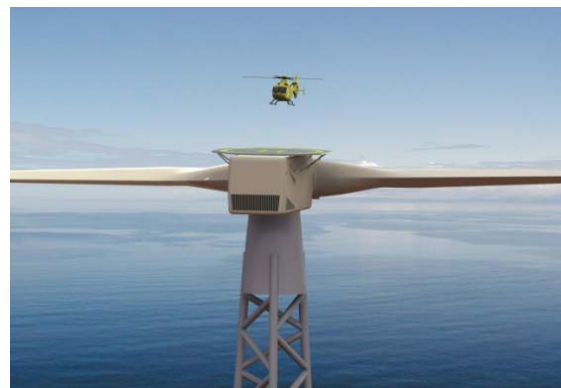
Figure 9: 2-blade offshore wind turbine (2B Energy)
