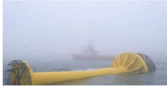
Figure 10: Float-out foundation (MBD Ocean Power)
